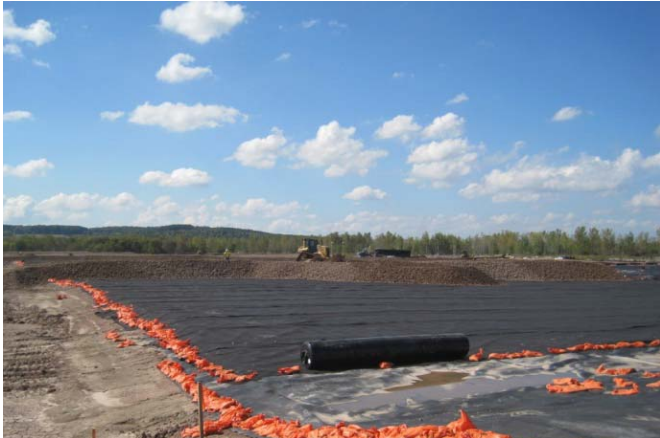
Installation of liner and drainage gravel
